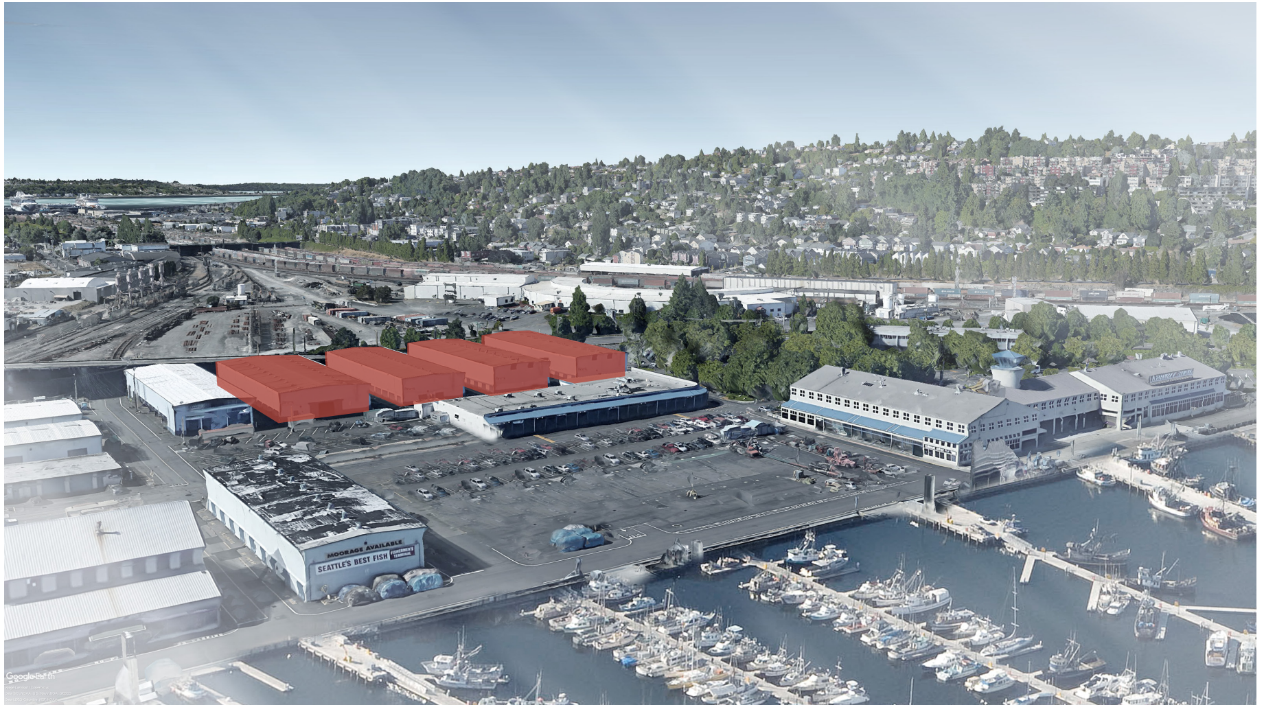
Figure 57. The four net sheds highlighted (Below) are full of solid fir dimensional lumber. At the time they were built, lumber was milled at larger dimensions than it is today. There is value in the sheer volume of material, and also in the antiquated cut of the wood. The wood itself develops properties over time, hardening from the weather and retaining the strength they had at the time of building. These changing properties are considered when reclaiming building materials for reuse, and lumber graders are given special training to accurately grade antique timbers.
