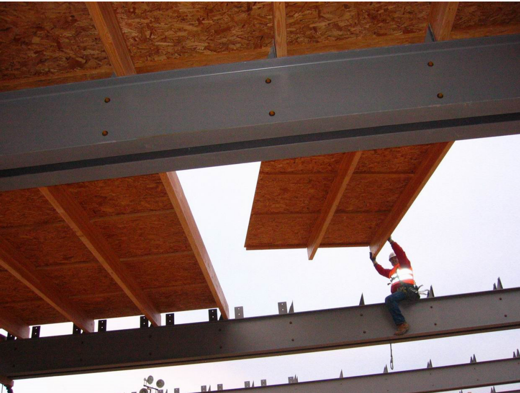
Figure 25. (Above). Panelized OSB and rafter assemblies being hoisted into place. This process took less than one day.
