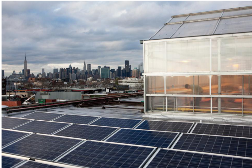
Fig. 17 | Rooftop Greenhouse in Brooklyn
