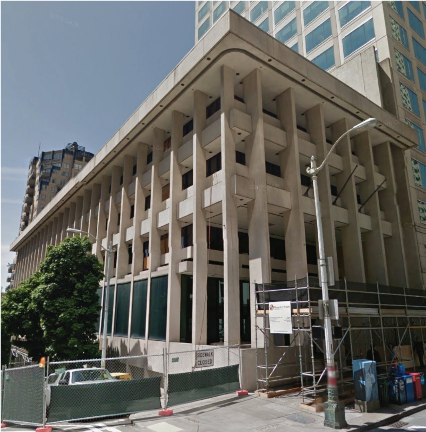
fig. 41 1101 2nd Ave. existing condition
