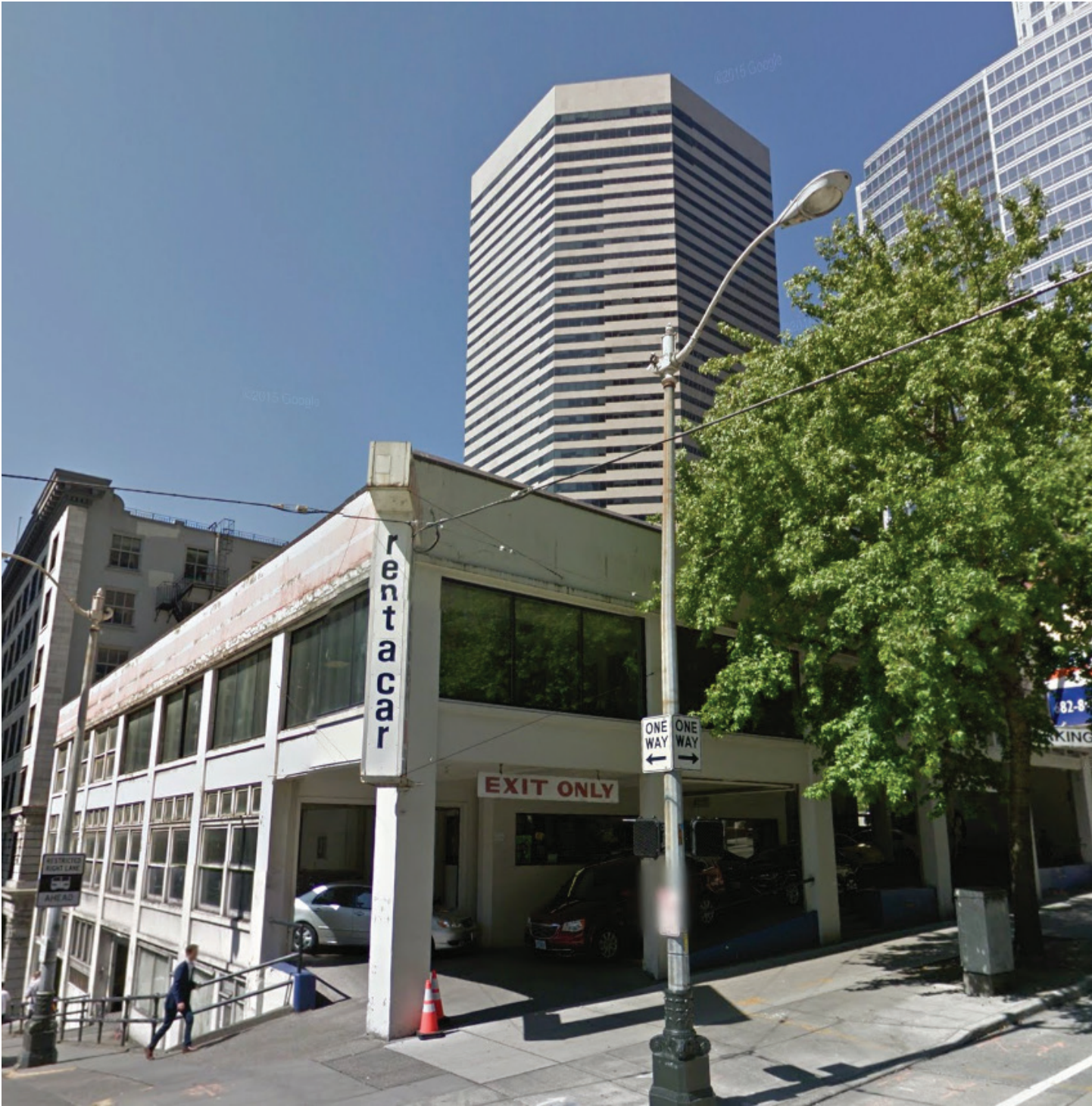
fig. 37 807 4th Ave. existing condition
