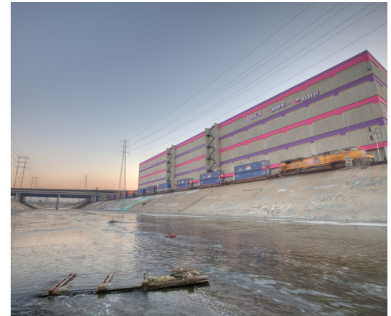
Figure 4. Distribution warehouse along Los Angeles River
